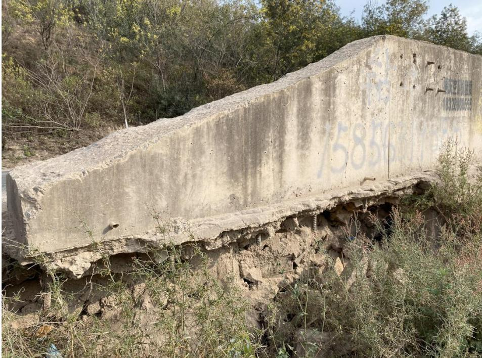
A photograph showing a large, weathered concrete retaining wall. The top edge of the wall is uneven and appears to be crumbling or broken. The wall is situated on a hillside with sparse vegetation. Blue graffiti, including the number '1585631988', is visible on the wall's surface.                                                                                                                                                               |
