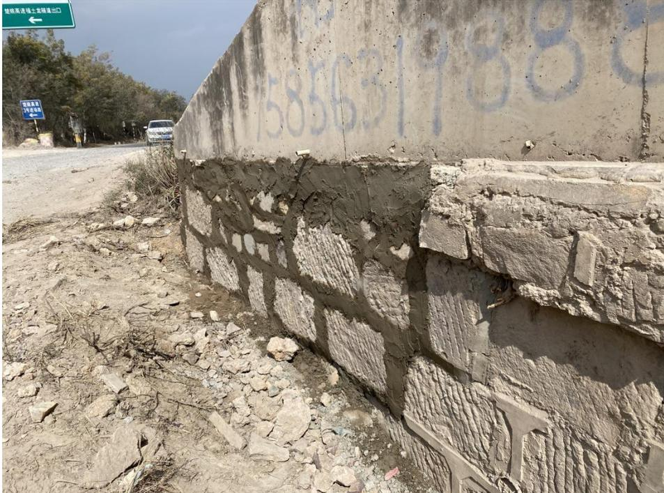
A photograph showing the same retaining wall after renovation. The top portion of the wall has been replaced with a new, more structured concrete structure. The lower portion of the wall is now constructed from large, rectangular stone blocks. The wall is situated on a dirt road with a green sign and a blue sign visible in the background. Blue graffiti, including the number '1585631988', is still visible on the upper part of the wall. |
