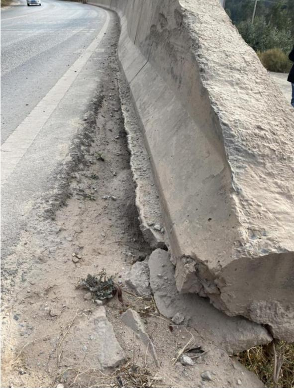
A photograph showing a concrete guardrail on the right side of a road. The guardrail is severely damaged, with large sections missing and the remaining structure crumbling. The ground around the base of the guardrail is loose soil and debris. The road surface is visible on the left side of the frame.                                |
